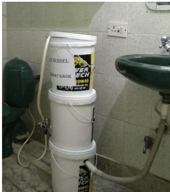
Figure 26: A photo of the installed setup demonstrates its ability to fit into a small space through vertical stacking.
