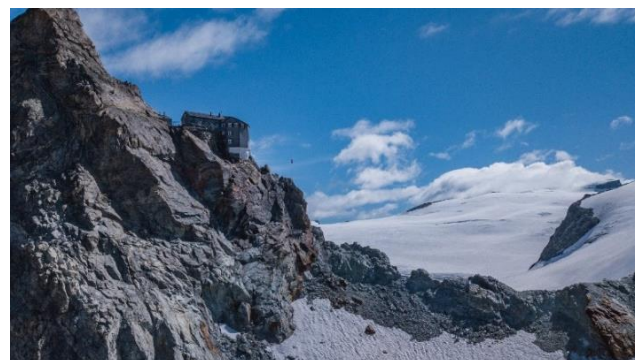
Figure 3 : The Bertol hut, in the centre of the image, on its rocky outcrop. The bell tower of the hut, also known as the Bertol bell tower, on the left, and the Bertol pass on the right. In the background, Tête Blanche (Source: Photo by Stéphane Schenk)
