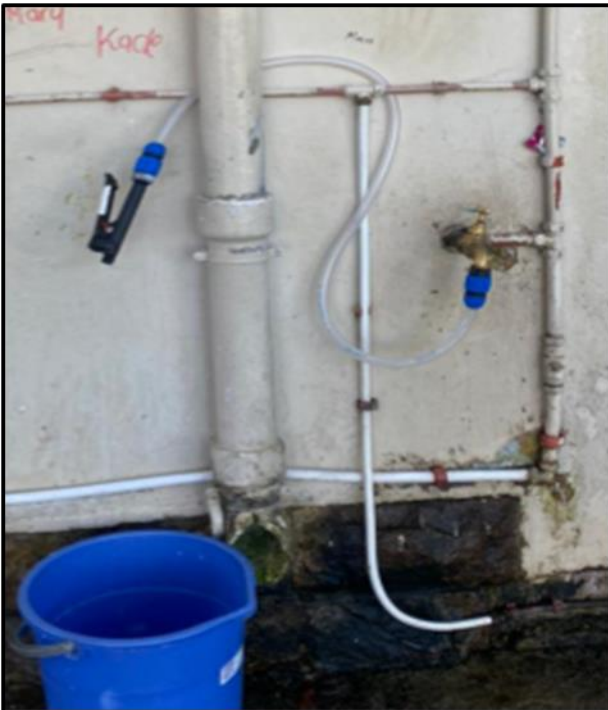
Figure 11: Our device installed at the leaking tap at our school.
