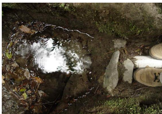
Example of a water seep
