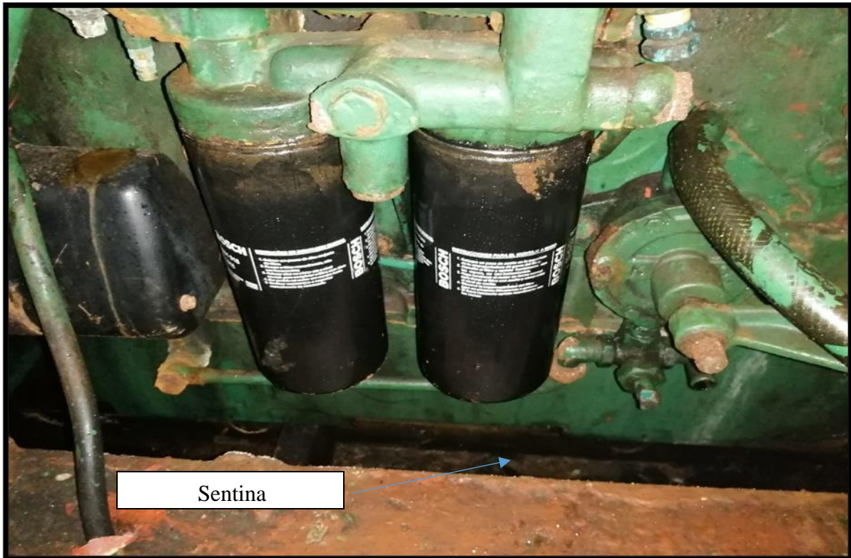
Image N°3 Filter and bilge system
