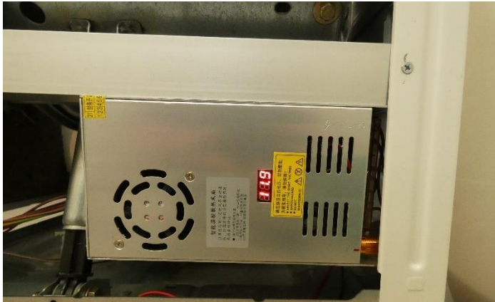
Figure 15 - shows the built-in power supply unit, view: right side of the washing machine, edge to the rear wall; photo: Luise Mast.
