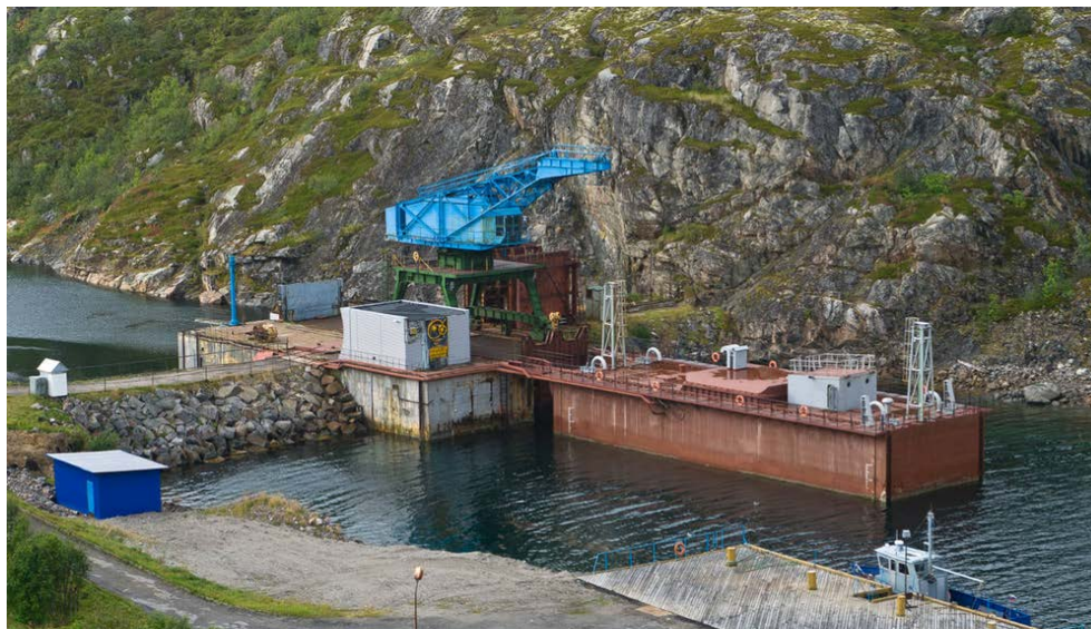
Fig. 2. Kislogubskaya tidal power station
