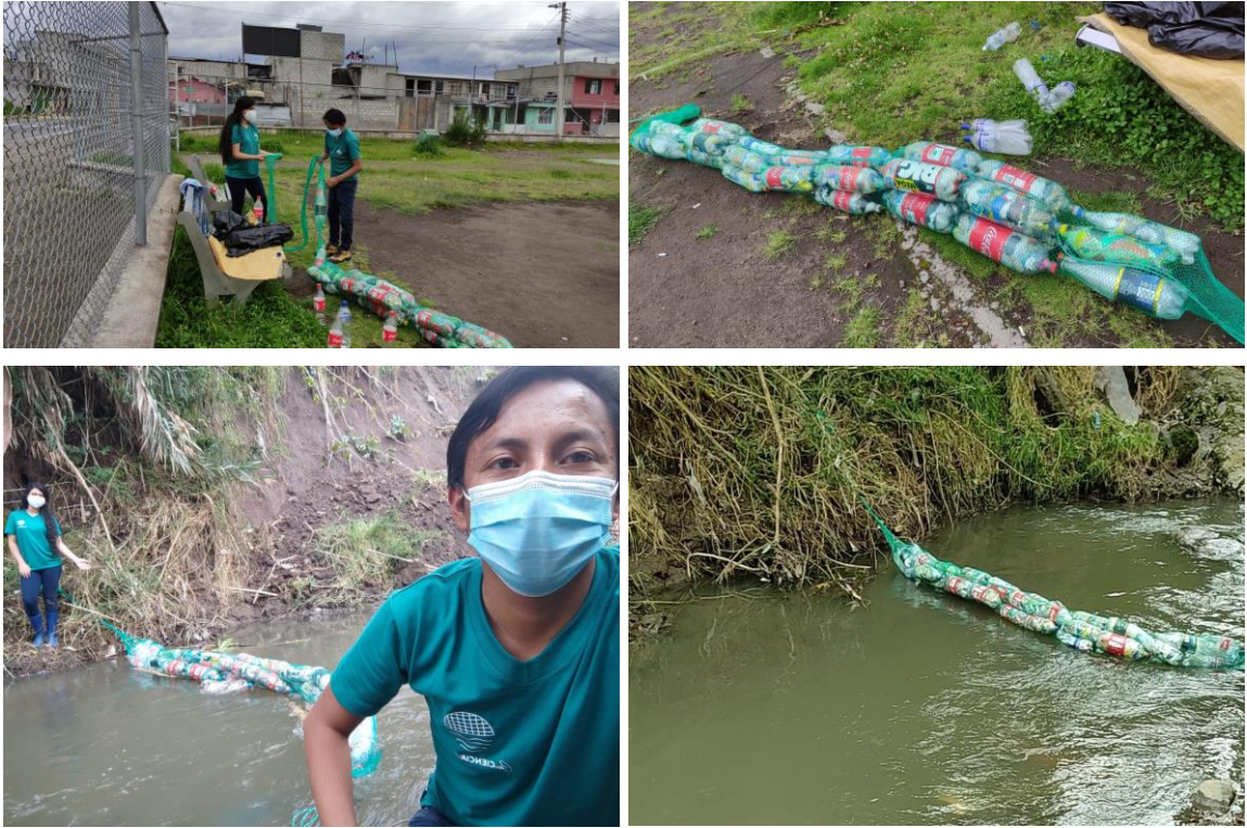
Illustration 6 . Elaboration of Ecobarda and implementation in the tributary of the Capelo River
