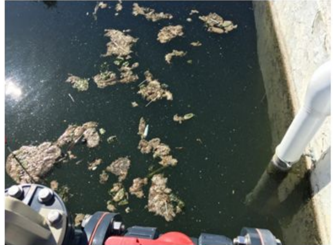
Figure 14 Image taken at Cobourg Water Pollution Control Department Treatment Plant #1, April 25, 2018: Feminine Tampon applicators and candy sticks are seen in the chlorine contact basin, the final step before the water reaches the effluent and out water bodies.
