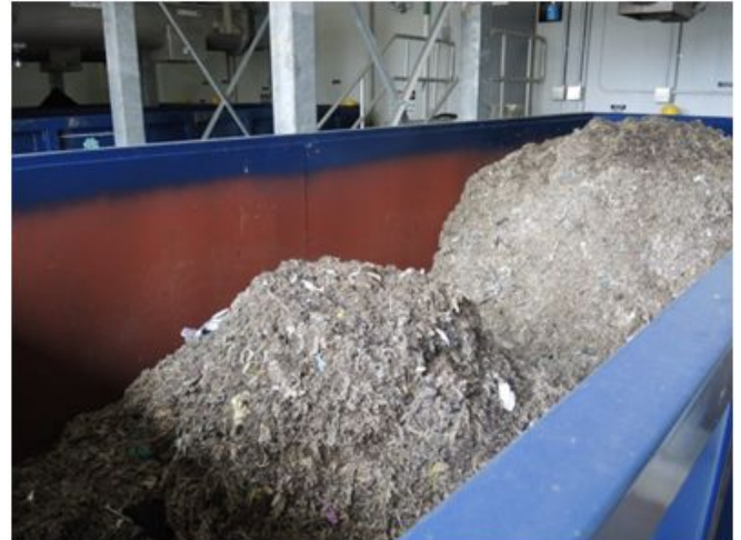
Figure 18 Image taken at Duffin Creek Water Pollution Control Plant, September 18, 2014: Non-flushable items, removed from the wastewater system, heading to landfill. Duffin Creek Wastewater alone sends one of these bins full every day.
