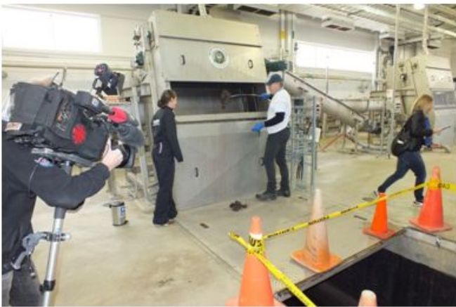
Figure 15 Image taken at Duffin Creek Water Pollution Control Plant, September 18, 2014: Barry Orr and I standing beside the Monster™ Finescreen Separation System, examining non-flushables clogging the screens.
